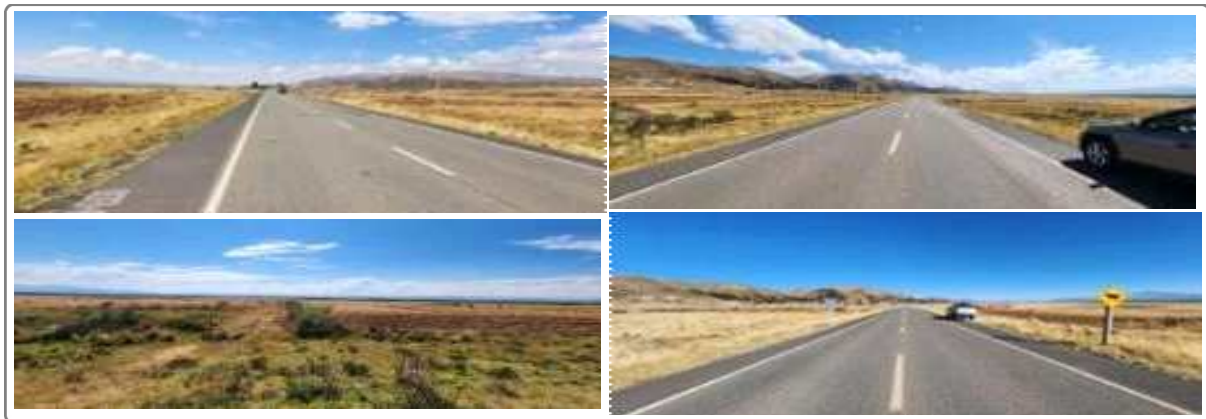
Figure 3. Field Survey Photos of Section 1
