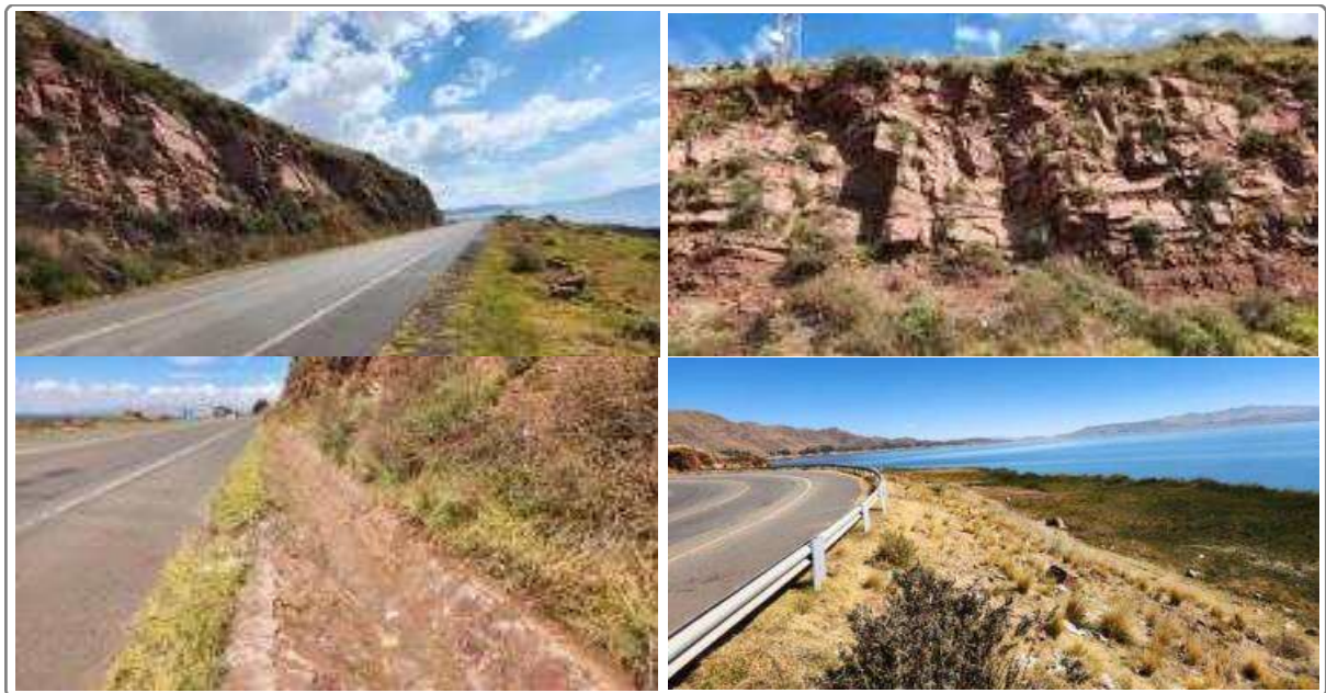
Figure 4. Field Survey Photos of Section 2
