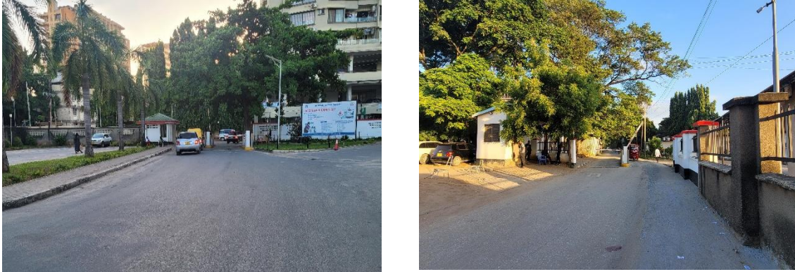
Figure 5. Current MNH-Upanga Infrastructure Picture.
